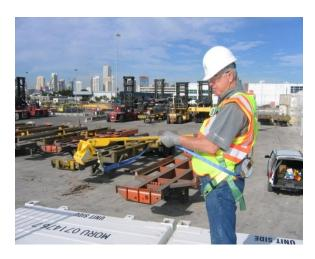
Extracting sufficient amount of webbing from SRL to allow worker to reach out and insert wand head into corner casting.
