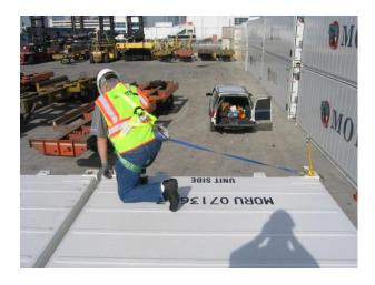
GM120 Top Lock Wand properly locked into corner casting and worker positioned correctly one container width away.
