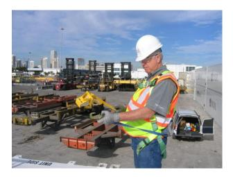
Connecting the double lock snap of the SRL to the anchor ring of GM120 Top Lock Wand.
